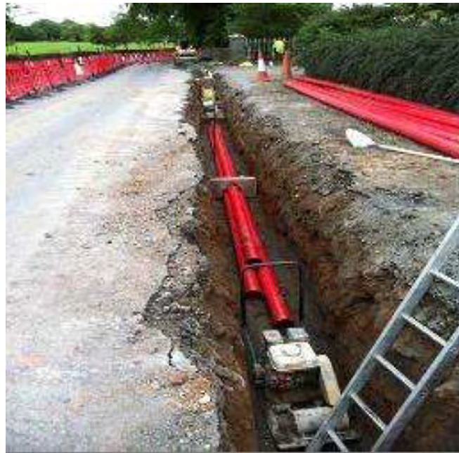
Image 2-1: Example of 110kV Underground Duct Installation
